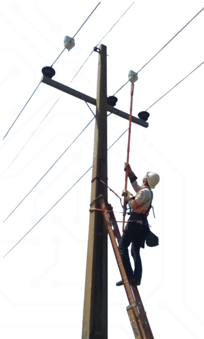
Figure 1: Installation using a ladder and a maneuvering pole, without the need to interrupt the power supply.
